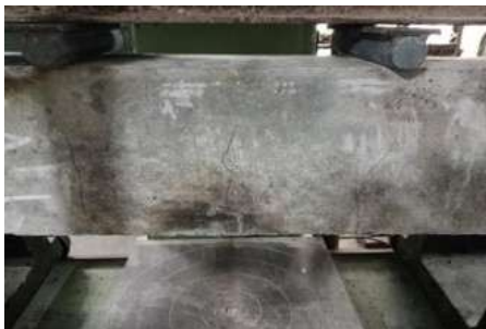
Fig.34 Failure crack pattern of beam with retardant additives (Combined Chitin & Metakaolin) subjected to fire
