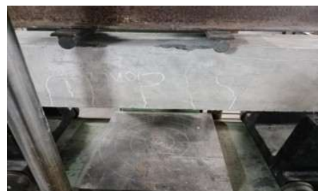
Fig.31 Failure crack pattern of control beam subjected to fire
