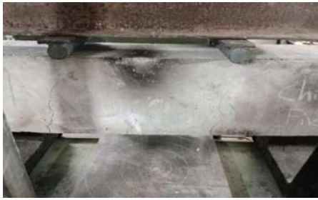
Fig.32 Failure crack pattern of beam with retardant additives (Chitin) subjected to fire
