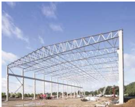
Fig. 1 Pratt Truss
