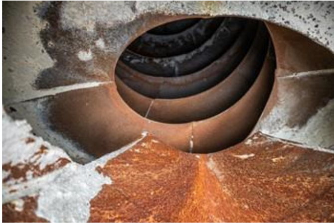
Figure 2. wear, tear and rusting on blade
