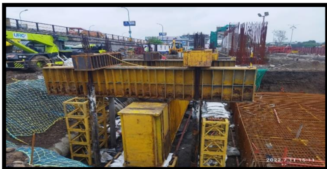
Fig. 9 alternate arrangement of initial load test on pile context of the equations, as well as the final solution to Res, and Raf
