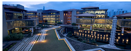
Fig-3: Suzlon energy building
