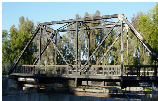
Fig. 1: Skeleton of a Typical Steel Truss Bridge
