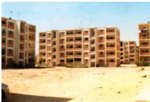
Figure.2 Lack of outdoor services in the public housing projects. Source: Author.
