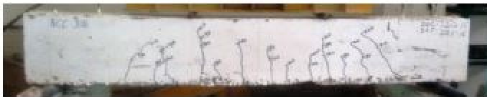
Fig. 6 CRACK PATTERN -III
