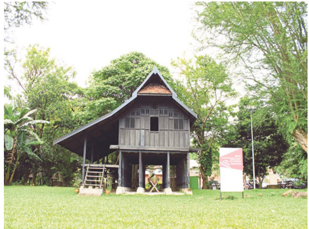
Figure 1.1: Example of Terengganu Traditional Malay House
