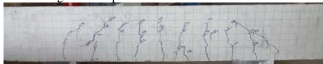
Fig.9. Crack pattern B-2
