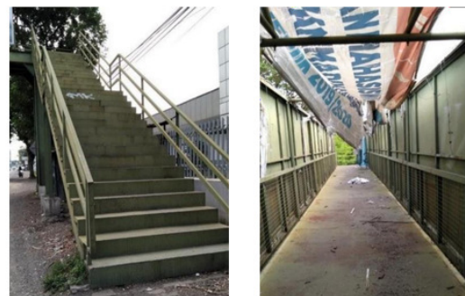
Figure 3. Steps and interior of the footbridge
