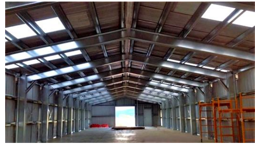
Fig .11. Cold formed steel warehouse in USA by McElroy METAL
