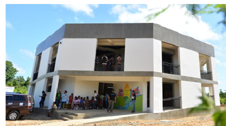
Figure 5. Multi-purpose Evacuation Center in Guiuan, Samar
