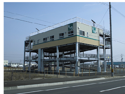
Figure 2. Tsunami Evacuation Tower Sendai City, Miyagi Prefecture
