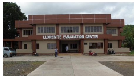
Figure 4. Llorente Evacuation Center
