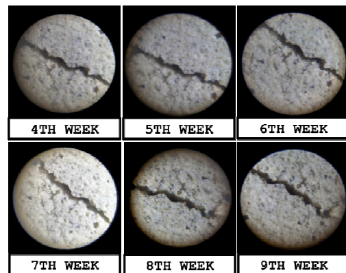
Fig. 1b. Visual observations of closure of cracks concrete with 7% bacteria
