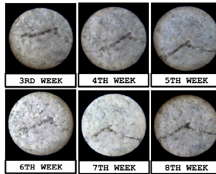
Fig. 2b. Visual observations of closure of cracks concrete with 7% bacteria
