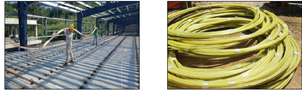
Fig. 1.1.g (left) shows on of the pioneer of the first distributors of GFRP bars in the Philippines and Fig. 1.1.h (right) shows the actual GFRP bars delivered in the construction site in Laguna. (Source: Armastek Philippines)
