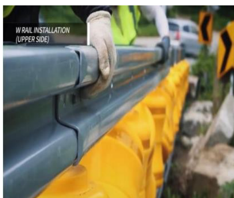
Fig. 5 W Rail Installation (Upper side)
