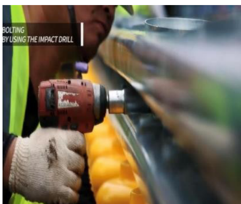
Fig. 6 Bolting by Using the Impact Drill
