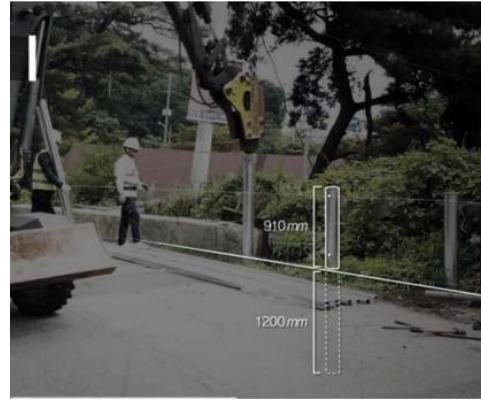
Fig 1 Main Post Installation
