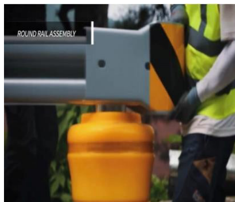
Fig. 8 Round Rail Assembly
