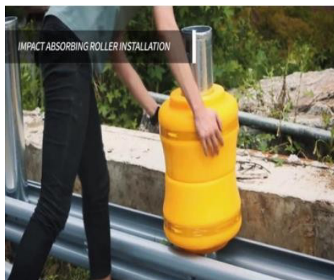
Fig. 4 Impact Absorbing Roller Installation
