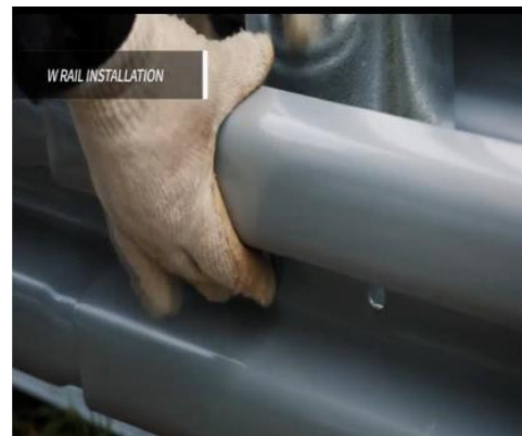
Fig. 2 W Rail Installation (Lower Side)
