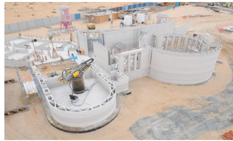
Fig-2: construction of building
