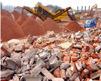
Fig. 2 Recycled aggregate concrete processing site
