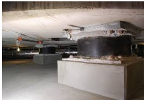
Base isolation frame structure
