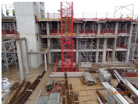
RCC frame structure
