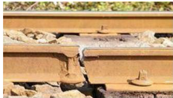
Figure. 1. Railway crack on track
